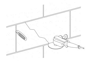
REMOVE ANY DEBRIS FROM THE ANCHOR CHANNELS OR SHIM
